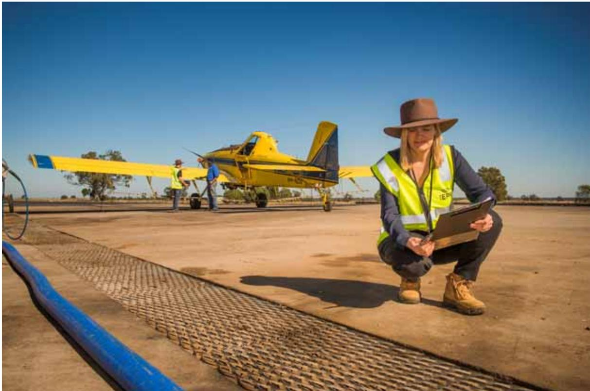
**Figure 7: Open drain covered with mesh to prevent solids entering the culvert
