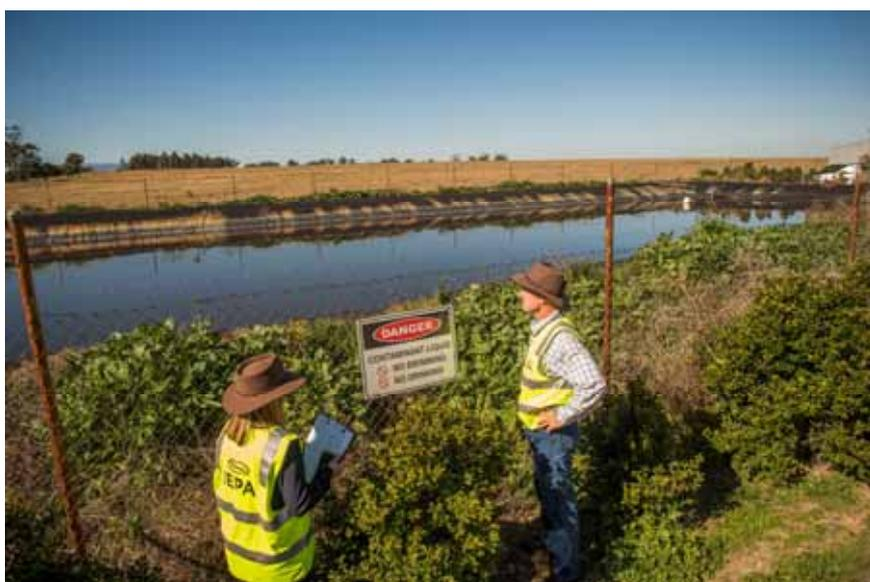
**Figure 4: Lined evaporation pond with signage and fencing**
