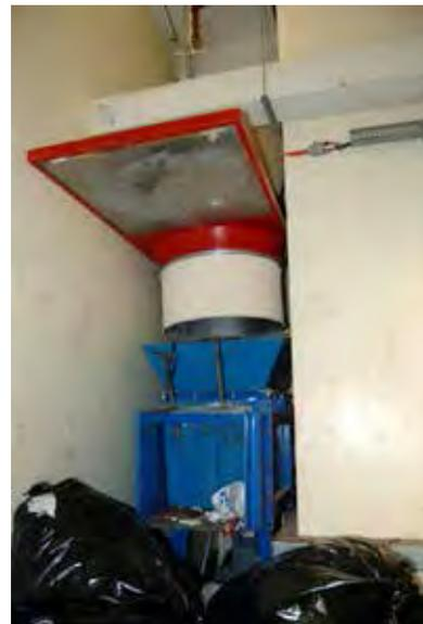
Figure 52 Compactor at chute base
