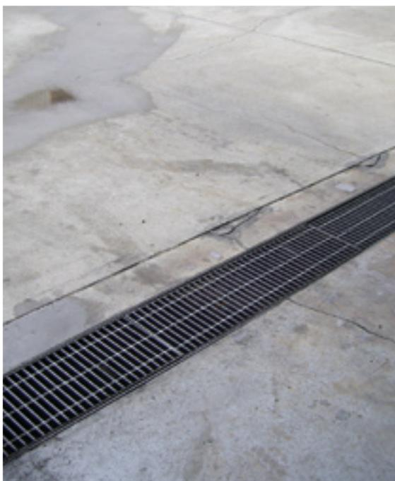
Bunded workshop with a grated drain that is connected to an oil/water separator.
