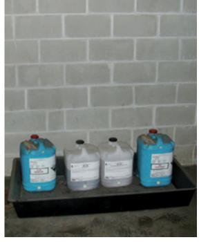
Another form of bunding is a spill tray, which is an effective solution for small containers and parts. Spill trays are available from industrial and safety products suppliers.
