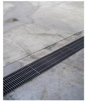
Bunded workshop with a grated drain that is connected to an oil/water separator.
