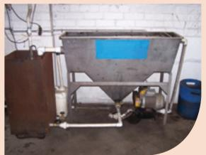
A coalescing (corrugated) plate interceptor (CPI) treats wastewater before it is discharged to the sewer.
