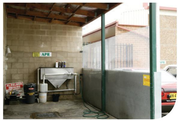
Conduct all washing in a wash bay with a collection pit. The pit should be connected to the sewer through an oil/water separator or to a storage tank.
