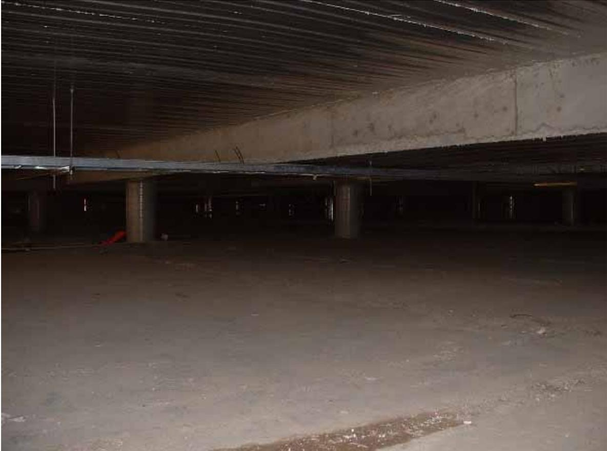
**Figure 8: Large vented sub-slab void**
