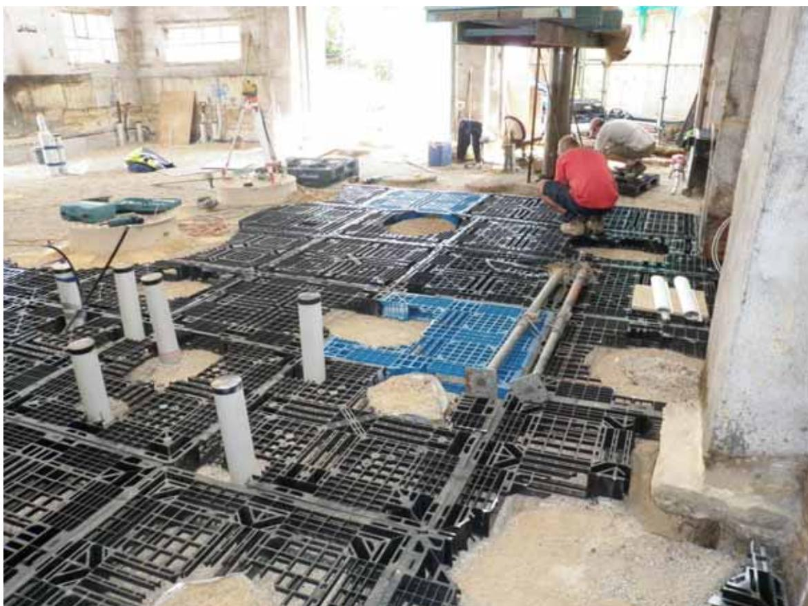
**Figure 7: Use of polypropylene formers to create a sub-slab void**
