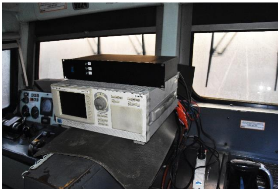
Power measurement device installed in-cabin
