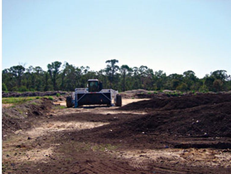
Figure 10. Straddle turner used to turn the compost windrows at the Hawkesbury City Council's Waste Management Facility.
