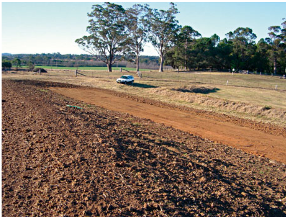
Figure 22. Area of CROA where vegetation and topsoil has been removed in preparation for the establishment of runoff plots (Blocks 2-4).
