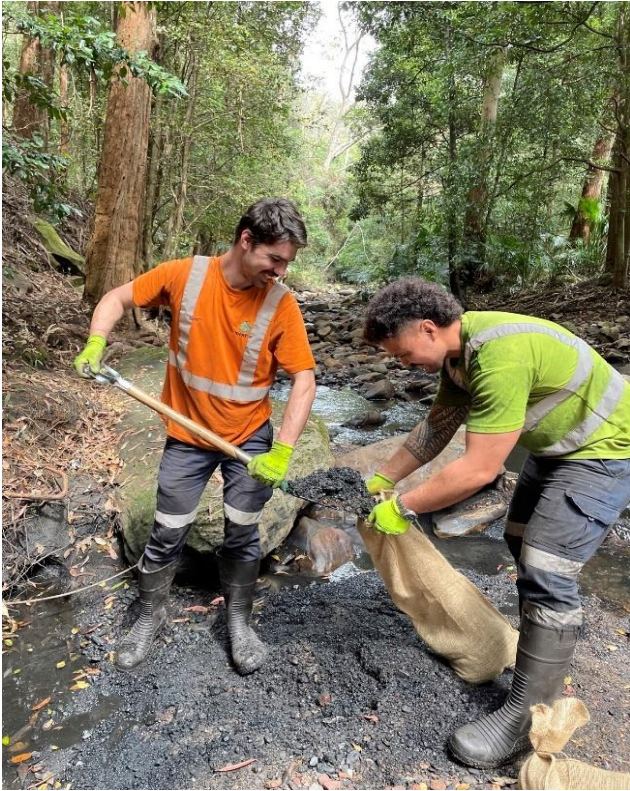
Photo 3.3 Work crew removing accumulated coal sediment from the creek floor
