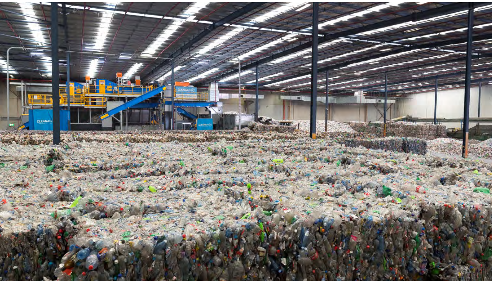
Cleanaway recycling facility at Eastern Creek which processes Return and Earn recyclables.
