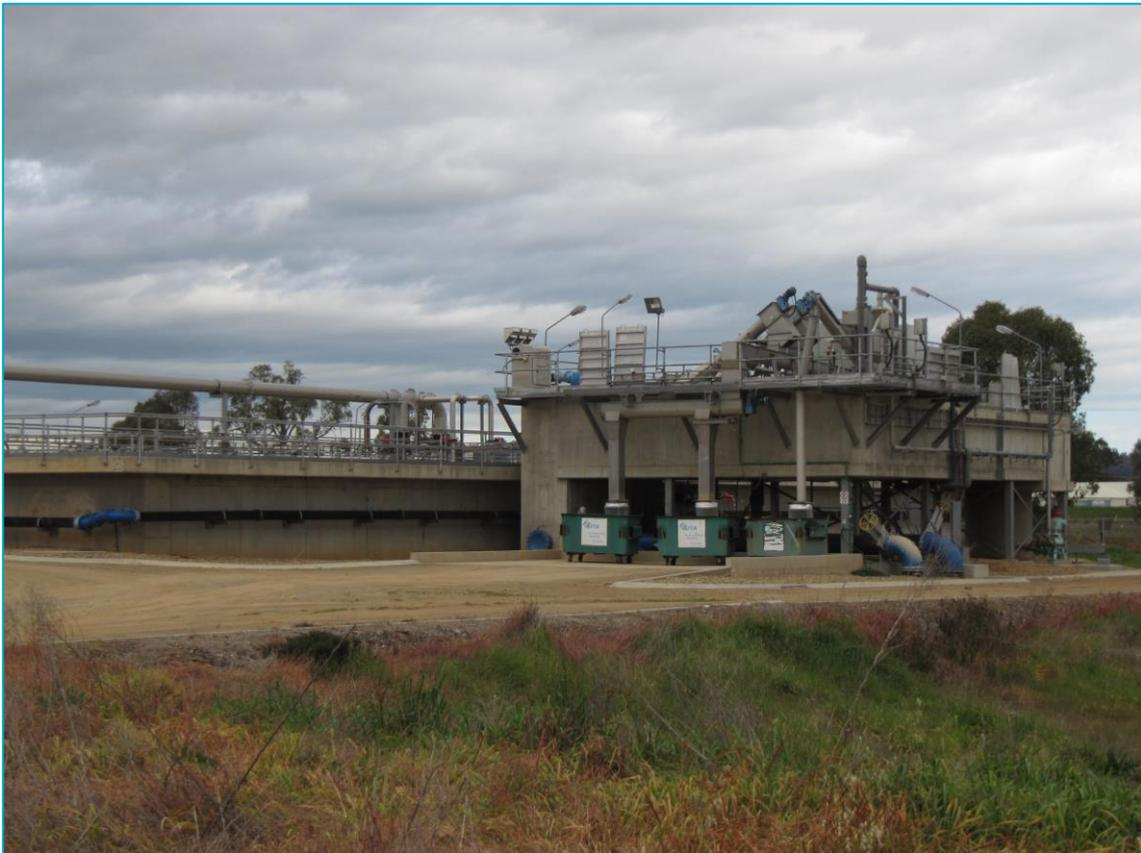
**Figure 6.42. Inlet of the newer treatment system at the Wagga Wagga facility. Note that the tanks are elevated above ground level.**
