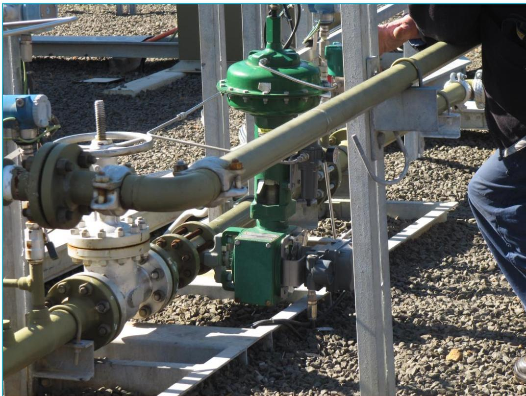
**Figure 6.24. Flow control valve and actuator on Well N1 (the green device in the centre of the photograph)**
