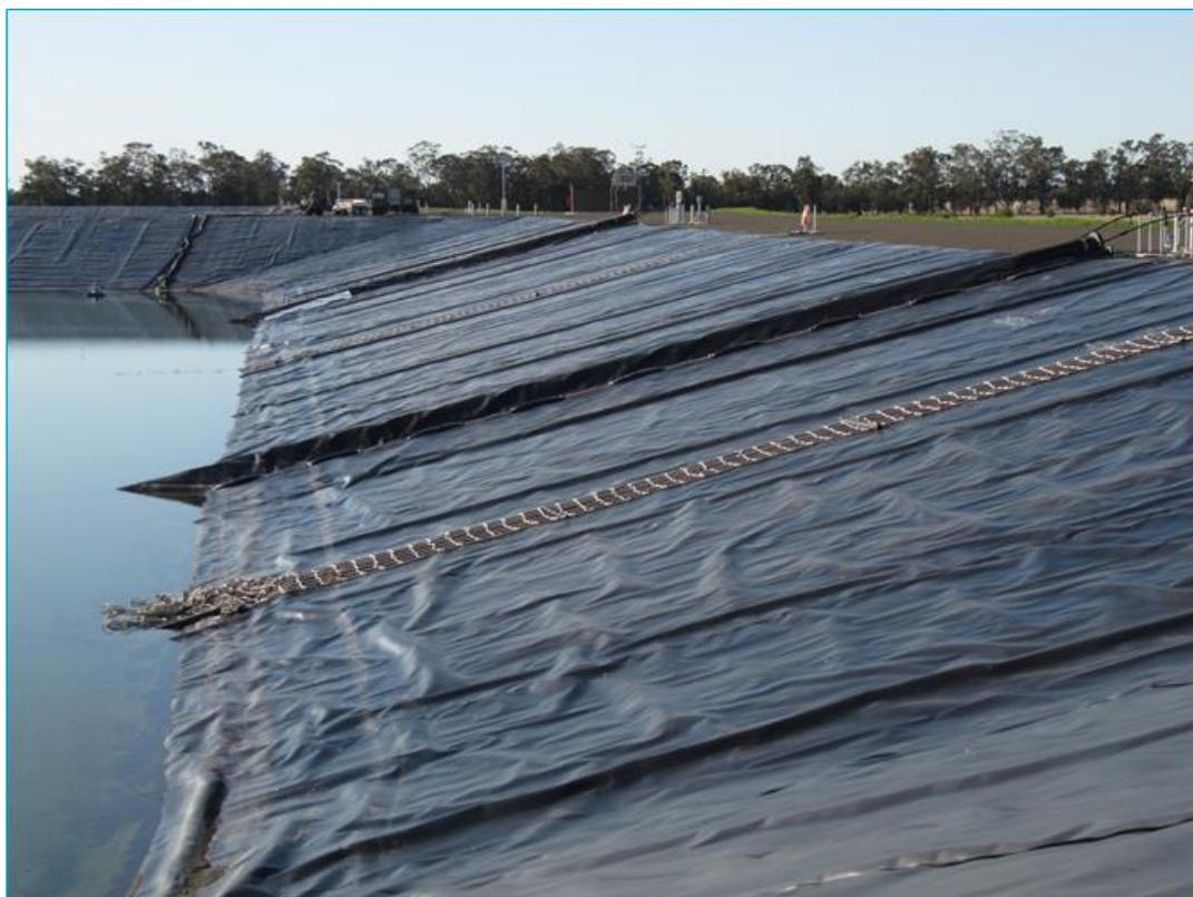
**Figure 6.25. Water retention pond at the Leewood facility in the Narrabri Gas Project. Note the rope ladders for accessing the water.**
