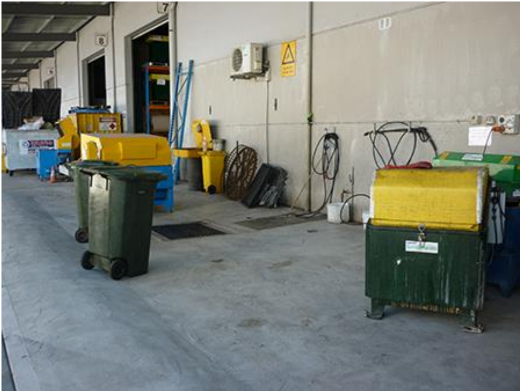
Good practice - liquid waste decanting area - rollover bund and roofed with blind sump
