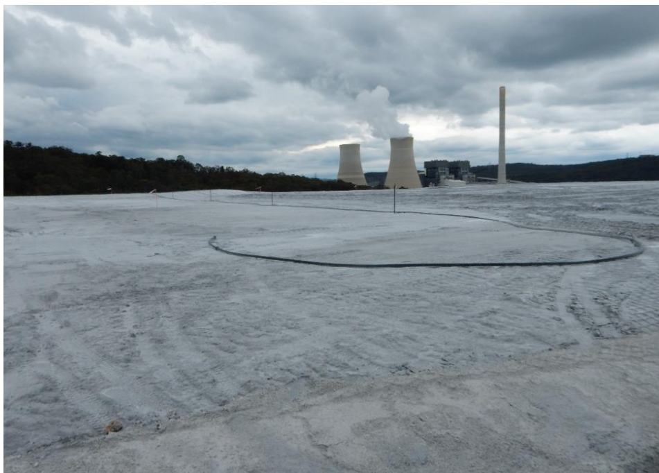
Figure 10: Dry ash emplacement with water sprays
