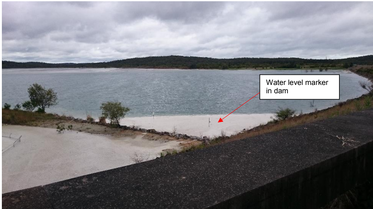
Figure 5: Coal ash dam with water level marker
