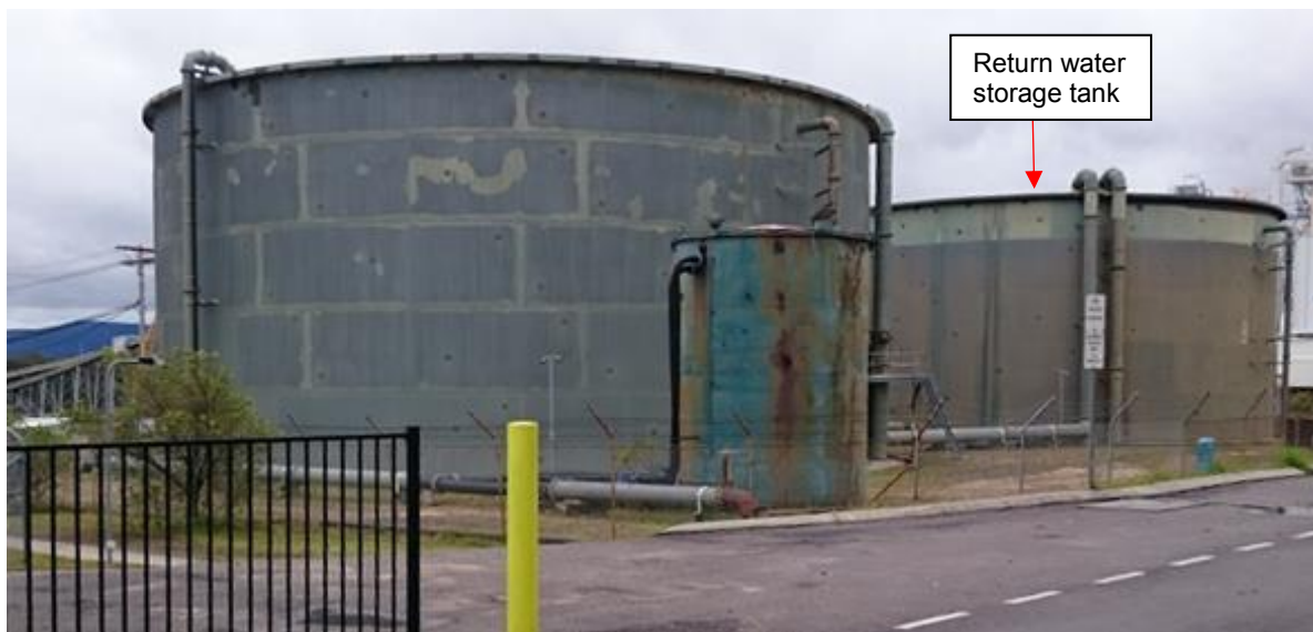
Figure 9: Return water storage tank in background without secondary containment (sewage tank is in foreground)
