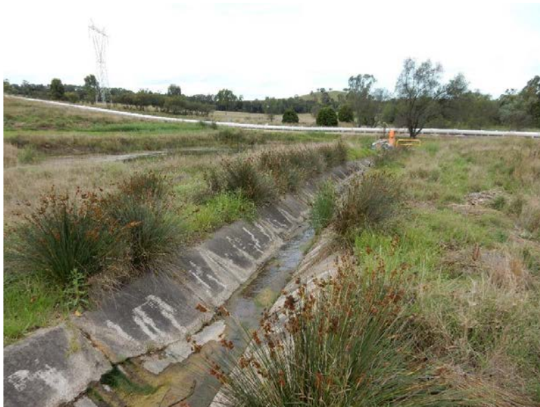
Figure 6: Seepage collection drain
