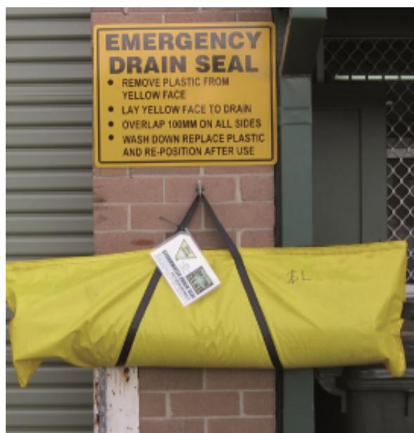
Clearly marked stormwater drain and raised door thresholds (left) and clearly marked spill response equipment to prevent spills entering drain (right).
