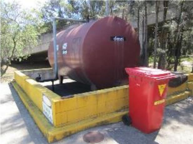
Large scale secondary containment solutions: bunding around storage tank
