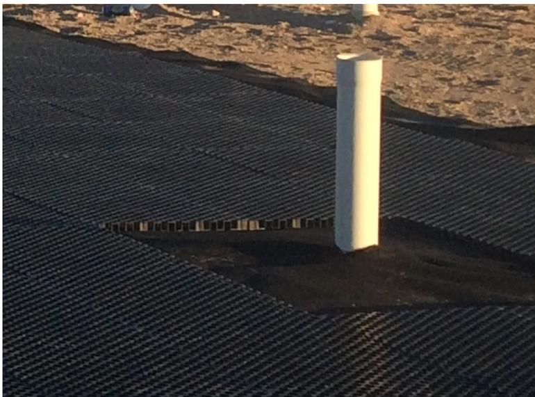
**Figure 8 Modular drainage system installed beneath membrane**
