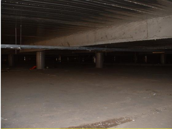
**Figure 9** Large vented sub-slab void
