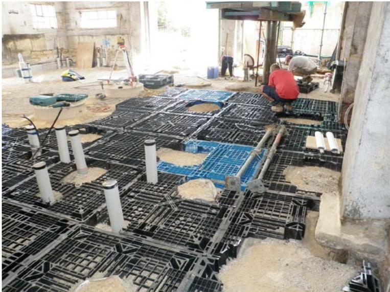
**Figure 7 Polypropylene formers create a sub-slab void**
