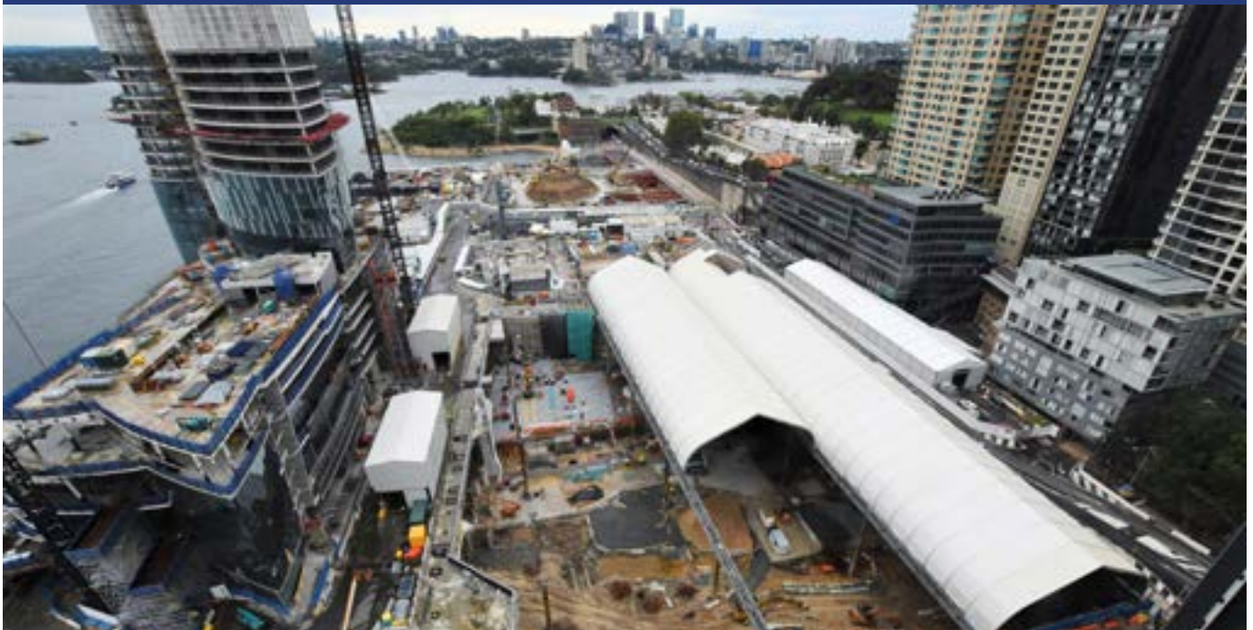
Tents (at right) help contain odours at the remediation site. Photo: Infrastructure NSW
