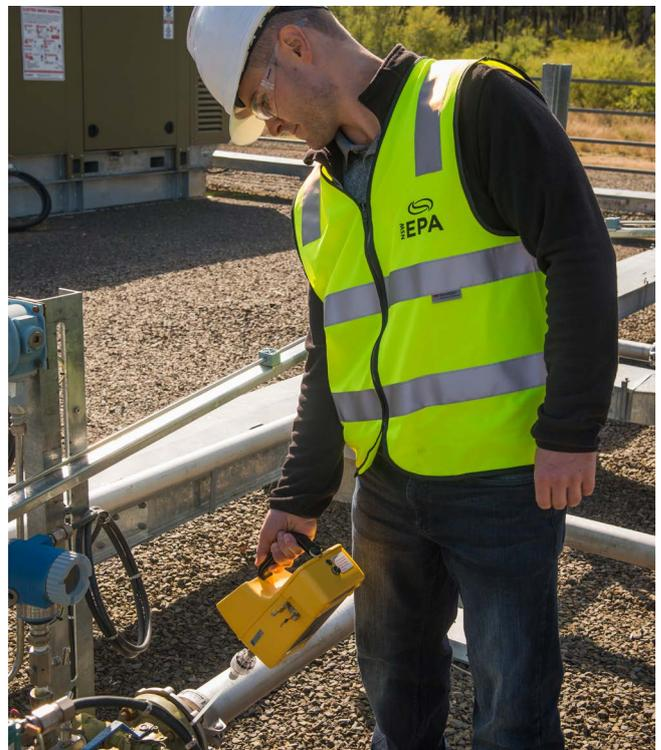
Leak Detection and Repair (LDAR) inspections are undertaken regularly by the NSW EPA at gas wells in NSW. Photo John Spencer/EPA.
