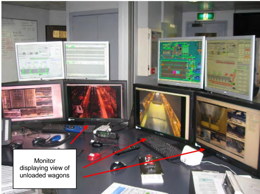
**Magnetic vibration device to dislodge hung up coal (top) and control room displays showing the interior of unloaded wagons to monitor for potential carry back coal (bottom) (photo: L Silk (top)/ R Deves (bottom))**
