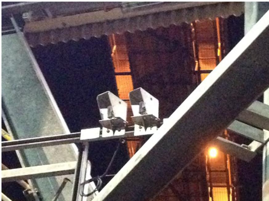
**Good practice: Fully automated loading at a load-out facility including control of the train speed from the control room (top) is achieved by tracking train movement by means of photoelectric cells (bottom) (photo: M Karam (top)/ T Greyling (bottom))**
