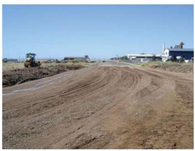
Photo 5. Recycled Sub-base ready for compaction
