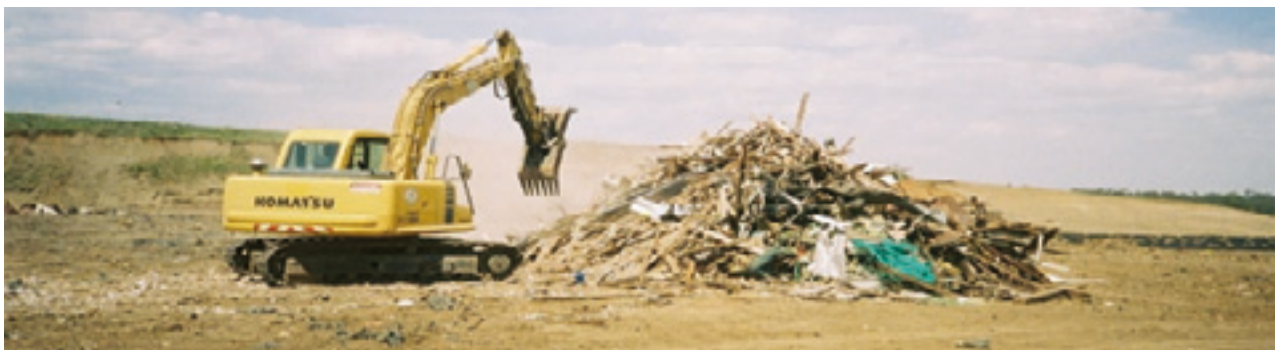
Photograph 1 – Mechanical mixing of large stockpile
