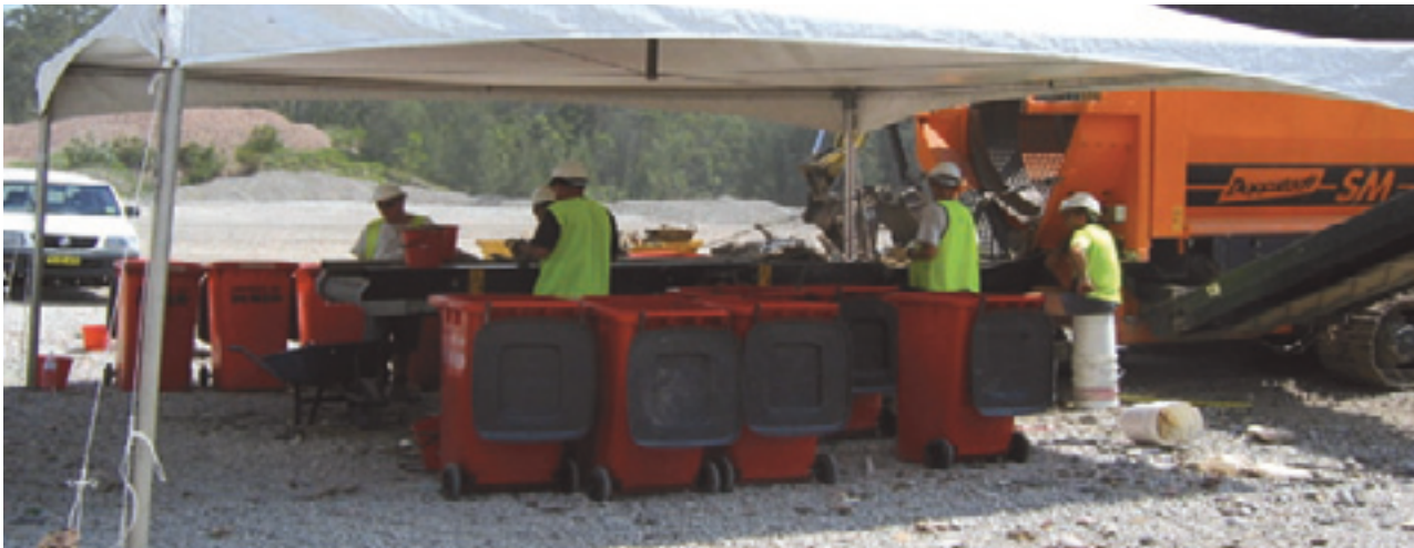
Photograph 2 – Doppelstadt trommel with picking belt, for manual sorting
