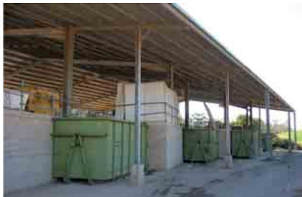
*Photo 21.4 Staggered arrangement of transfer station bins*
