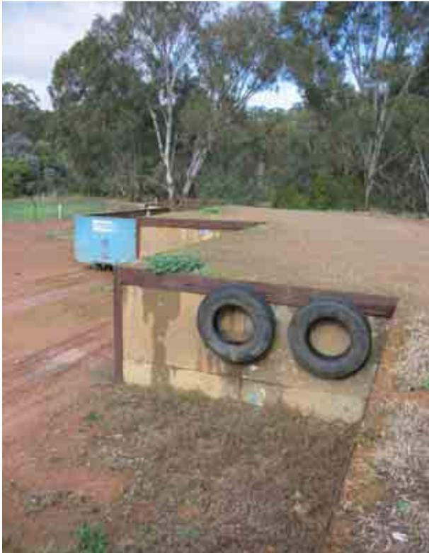
Photo 17.1 Staged platform arrangement, no safety barriers
