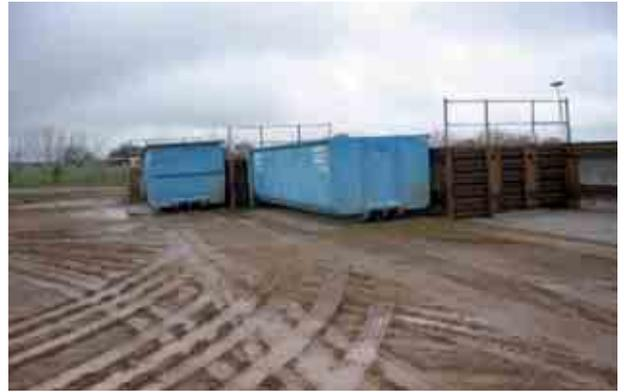
*Photo 16.3 Cement base under transfer bins, concrete and steel reinforced retaining walls*
