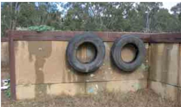
Photo 17.2 Tyres used for protection of the platform retaining wall
