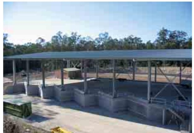
Photo 24.5 Saw tooth arrangement
