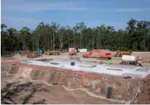
Photo 24.15 Construction of the waste transfer station platform
