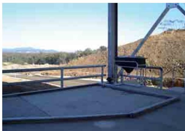
Photo 24.14 New bunded area on platform for lead acid batteries and waste oil
