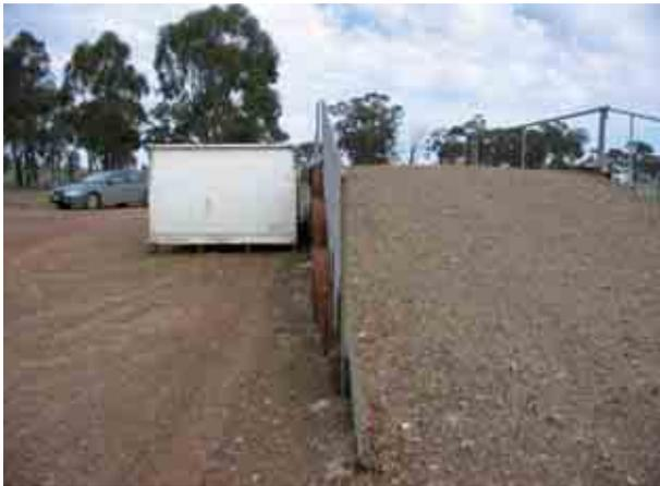
*Photo 18.2 Single ramp up and down to single skip bin*
