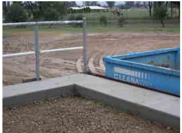
*Photo 16.4 Concrete lip to prevent vehicles backing over the platform edge*
