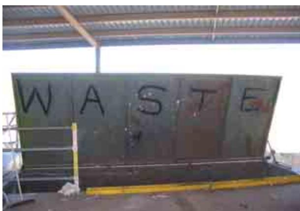
*Photo 21.3 Insufficient barriers to prevent falls into transfer station skips*
