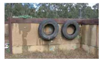
Photo 17.2 Tyres used for protection of the platform retaining wall
