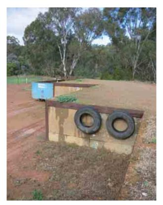
Photo 17.1 Stagged platform arrangement, no safety barriers
