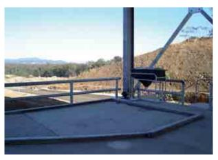
Photo 24.14 New bunded area on platform for lead acid batteries and waste oil
