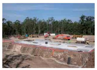
Photo 24.15 Construction of the waste transfer station platform
