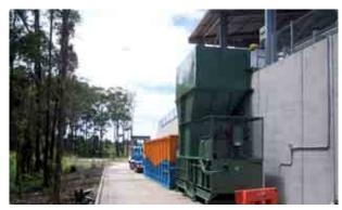
Photo 14.5 Stationary compactor and transfer container
