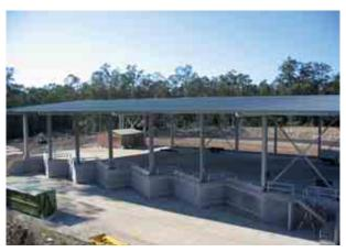
Photo 24.5 Saw tooth arrangement
