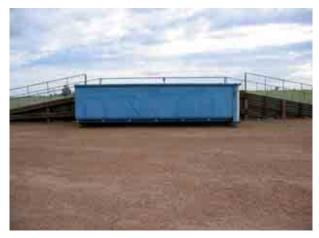
Photo 18.1 Single skip bin, ramp with hand rails
