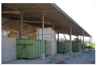
Photo 21.4 Staggered arrangement of transfer station bins
