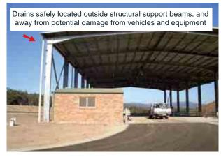
Photo 24.9 Location of drainage pipes
