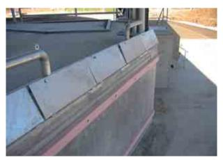
Photo 24.6 Platform edge, safety rails and hardwood buffers
