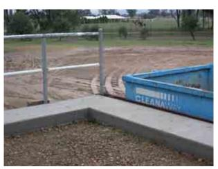
Photo 16.4 Concrete lip to prevent vehicles backing over the platform edge
