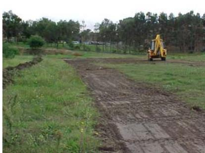
**Plate 8.** Site preparation. Grass was removed from the surface of the site and formed into berms to prevent runoff.
