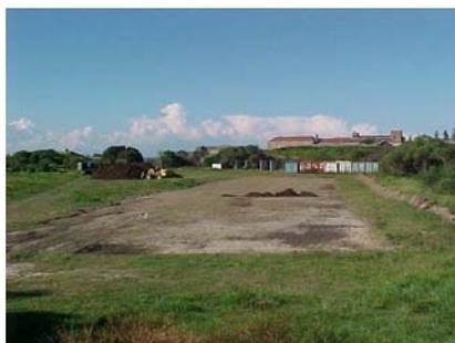
**Plate 9.** Site established. A loader formed the nine static piles with a berm of compostable organics between each treatment to prevent cross-contamination.
