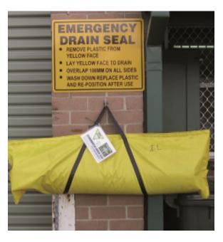
Clearly marked stormwater drain and raised door thresholds (left) and clearly marked spill response equipment to prevent spills entering drain (right).
