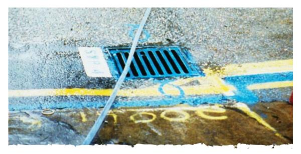
Do not place hoses over stormwater inlets (DECC)
