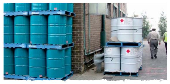
Chemicals should not be stored close to stormwater inlets (DECC)
