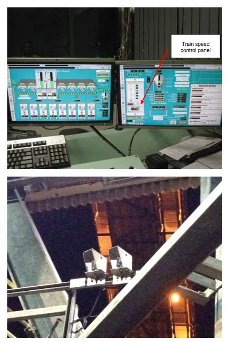
Good practice: Fully automated loading at a load-out facility including control of the train speed from the control room (top) is achieved by tracking train movement by means of photoelectric cells (bottom) (photo: M Karam (top)/ T Greyling (bottom))
