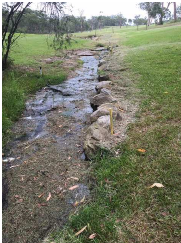
Photograph 2: Drainage from the golf course flowing to Ourimbah State Forest
