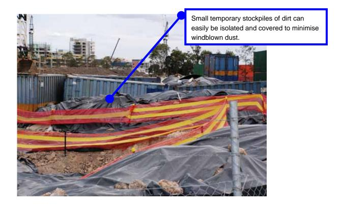
Dust from a large construction site like this one can be transported off site on the wheels of any vehicles moving out of the site. Dirt and mud deposited on surrounding roads will be pulverized into fine dust by traffic and then present a real nuisance to neighbours.
