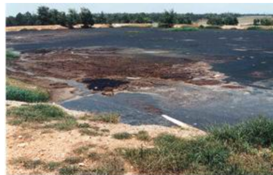
An overloaded effluent pond
