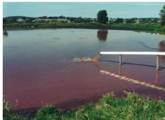
An effective effluent pond—the pink colour indicates bacterial activity
