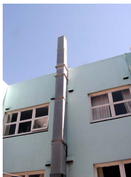
This take away food shop is on the ground floor of a three-storey block of flats; the odours are vented through a high stack above a small courtyard.
