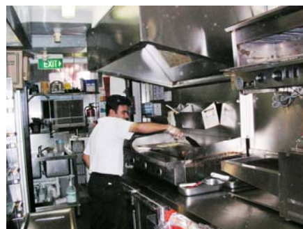
This take away food shop is on the ground floor of a three-storey block of flats; the odours are vented through a high stack above a small courtyard.
