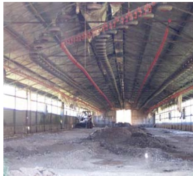
Removing waste litter in a large poultry shed
