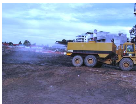
Using water and surfactant sprays to suppress dust
