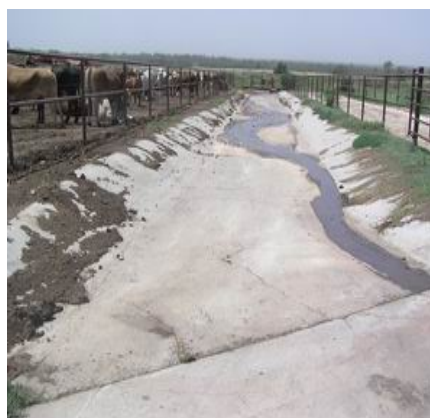
Well-constructed self cleaning concrete drain at a feedlot
