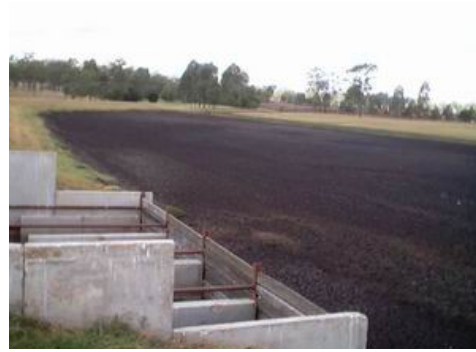
Dry sedimentation basin showing weir to effluent holding pond
