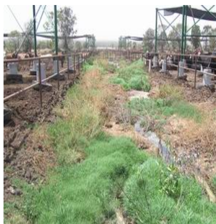
Poorly maintained drain— weeds and manure build-up
