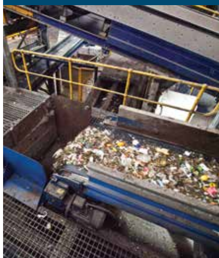
Global Renewables UR-3R waste facility recovering materials for recycling.
