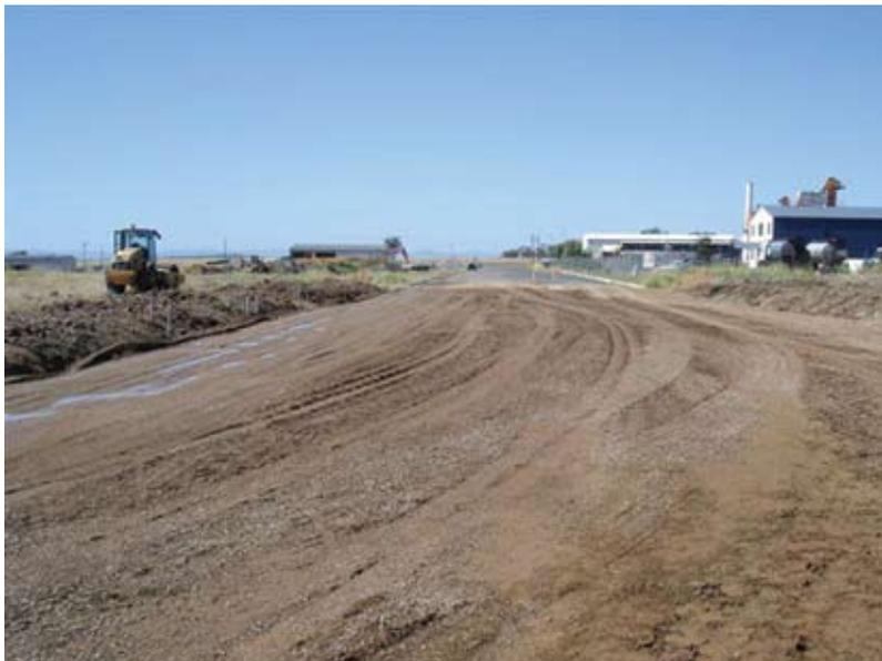
*Photo 5. Recycled Sub-base ready for compaction*
