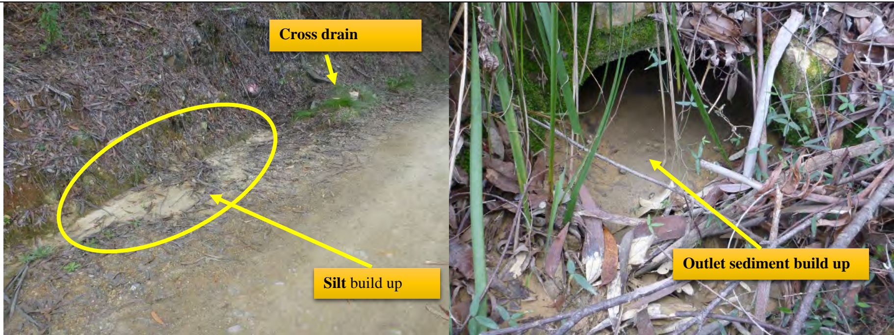
Figure 19: Cross drain entrance inlet, and outlet showing considerable sediment build up.
