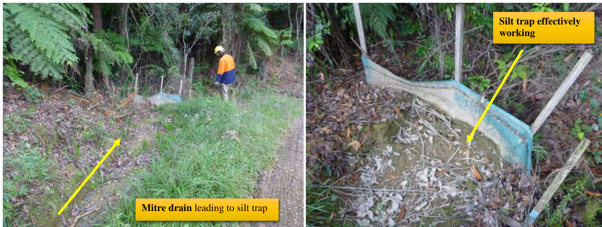
Figure 18: Mitre drain leading to silt trap, with silt build up
