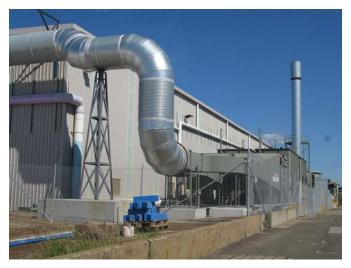
Temporary emission control enclosure, former Orica chlor alkali plant/M Hart, EPA
