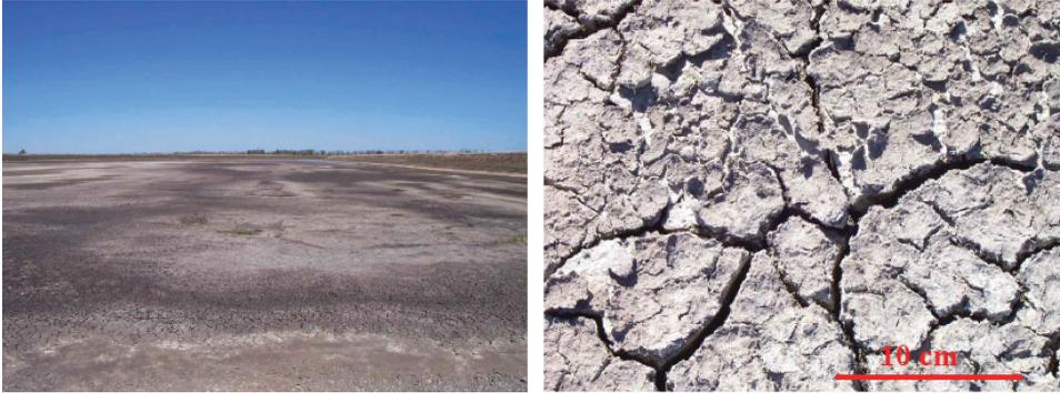
**FIGURE 4.** Evaporation ponds at Dalby (QLD) showing evidence of cracking.<sup>101</sup>
